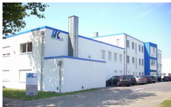
STI Head Office Duisburg, Germany
